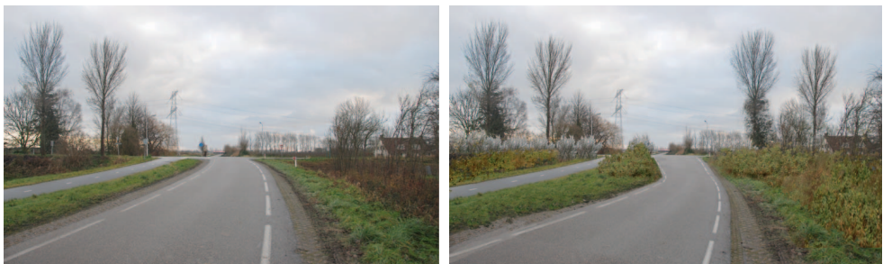
Fig. 7. Dangerous intersection of a road not situated on a dike with a dike road (on the background). Left: In the present situation the road in front leads fluently to the dike road, making the dike invisible. Right: The proposed solution is to accentuate the characteristics of the dike road by planting trees on the dike and a less fluent bend with a sharper slope of the other road (Van Blerck et al., 2009).
